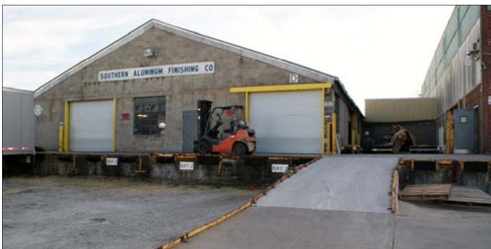
Building D 21,075 SF
